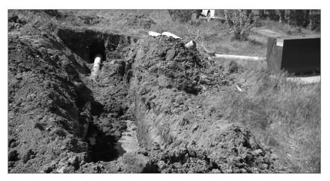
A dig-in by a customer replacing their water line without locates. The UG transformer in the upper right had underground lines directly where the customer dug with a backhoe. Luckily, no one was injured. It was a dangerous and costly mistake for the customer.
